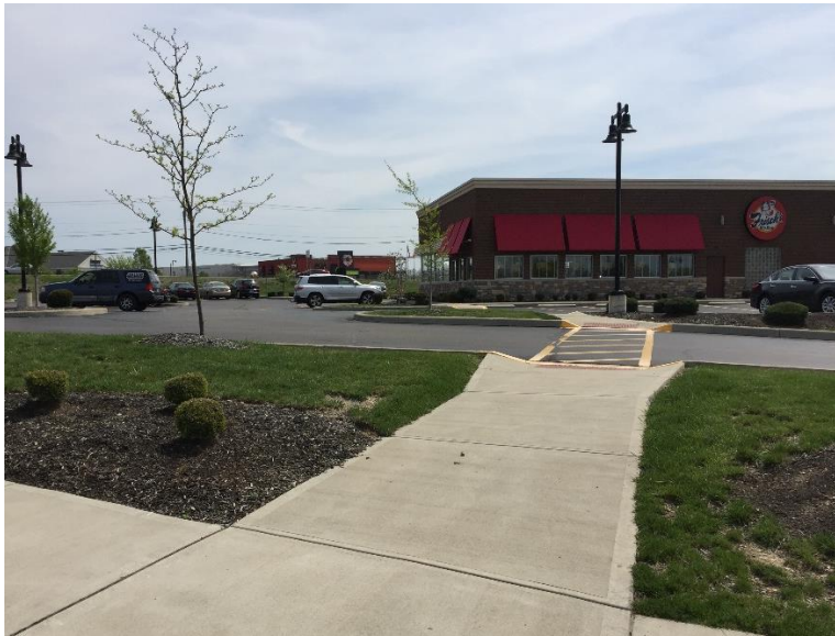
Figure 7.3-1: This image illustrates a sidewalk connection between a building and a public sidewalk in the right-of-way. This connection includes both a separate sidewalk (foreground) and a connection delineated through a painted line (background).
