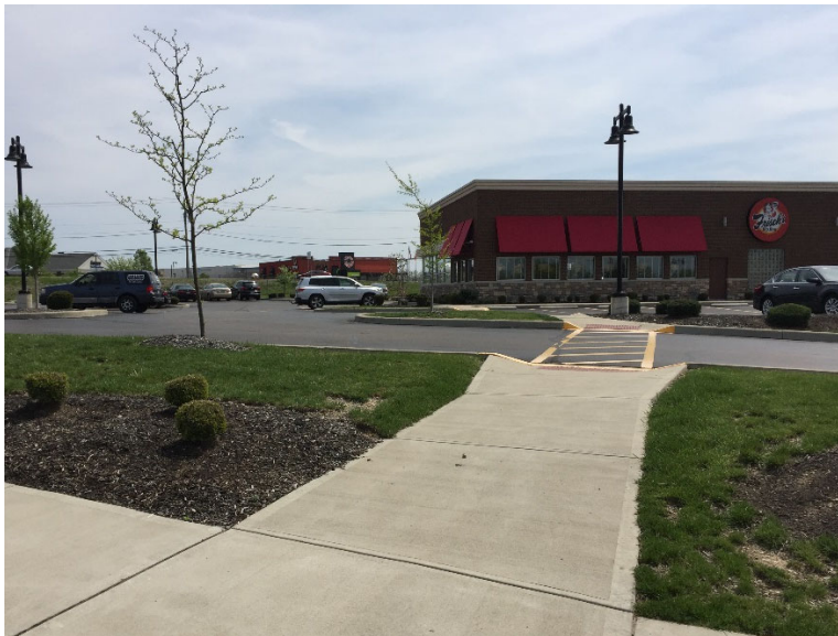
Figure 7.3-1: This image illustrates a sidewalk connection between a building and a public sidewalk in the right-of-way. This connection includes both a separate sidewalk (foreground) and a connection delineated through a painted line (background).
