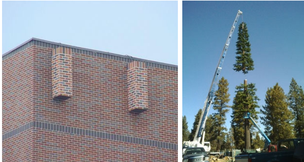
Figure 4.9: Examples of Stealth Designs for Telecommunications Towers
