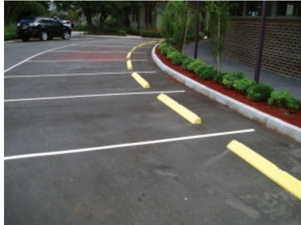
Figure 7.6-4: Wheel stops or continuous curbs shall be setback two (2) feet from pedestrian walkways to prevent vehicles from driving onto the walkways. Where both wheel stops and continuous curbs are present, the two (2) feet shall be measured from the wheel stops.
