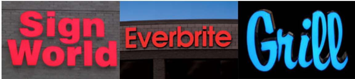
Figure 11.2-7: Illustration of a channel letter sign.
