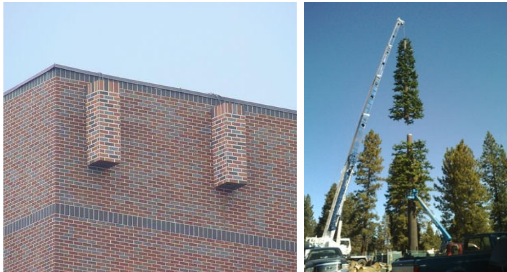
Figure 4.9: Examples of Stealth Designs for Telecommunications Towers
