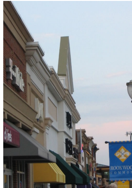
Figure 6.1-2: The image on the left illustrates the use of parapet walls to screen mechanical equipment. Tall, thin parapets such as the one shown in the image on the right should be avoided to prevent the appearance of false walls.
