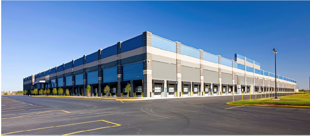
Figure 6.2-1: Illustration of how the façade design requirements such as columns may be applied to industrial buildings.
