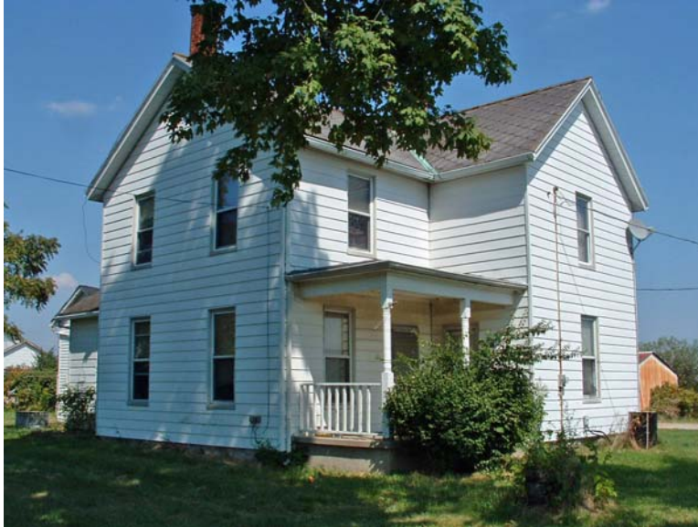
61. 8000 Hamilton Mason Road, parcel D2010-009.000-007 Constructed in 1900, Ross residence/Gorsuch farm/owner by Hen-Jur LLC
