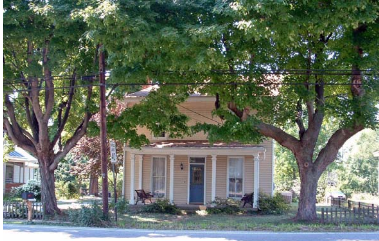
50. 6491 Cincinnati Dayton Road, parcel D2030-050.000-039 McClung/Allen/James Ray and Dessie M. Bolin house (built c. 1846 – 1853) interesting story about the WPA concrete out house.
