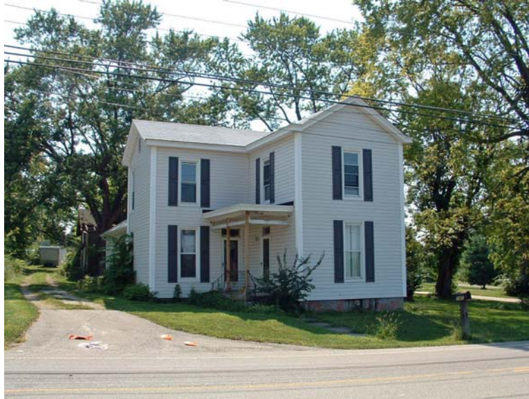
43. 7485 Princeton Road, parcel D2030-049.000-033 Constructed in 1869, Anderson/Chance/David H. Cradler home
