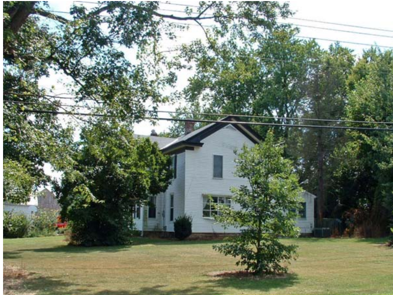
24. 6237 Kyles Station Road, parcel D2010-023.000-007 Constructed in late 1800, tied to Osman family, owned by Judy M. Allie
