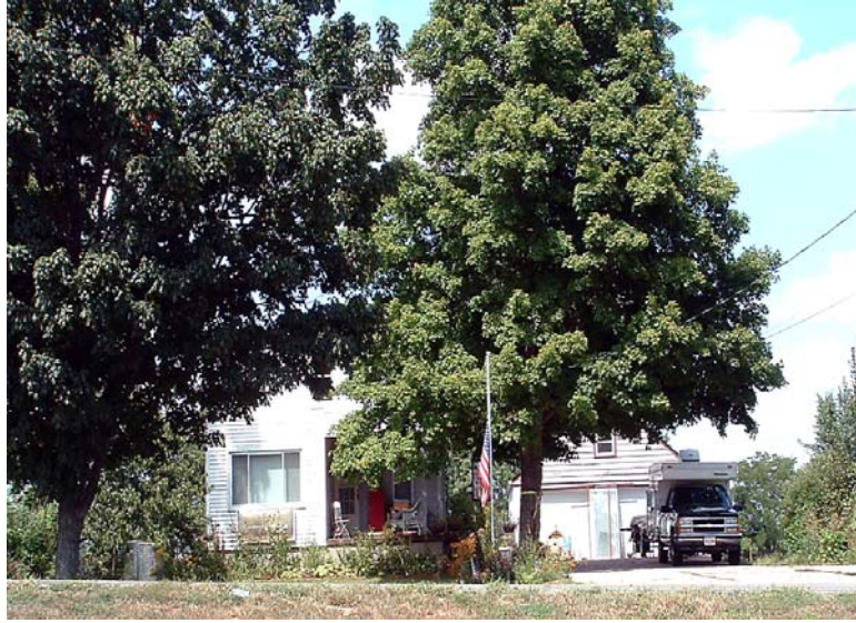
19. 4842 Millikin Road, D2020-031.000-004 Constructed in 1926, Penny D. and Robert J. Gibson Residence
