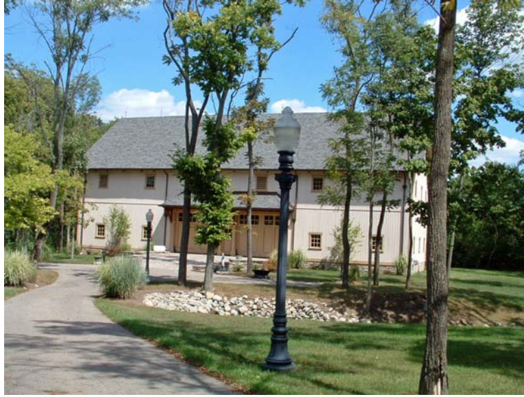
11. 6312 Princeton Road, restored historical barn owned by Marc T. and Nancy Terry, D2010-002.000-036
